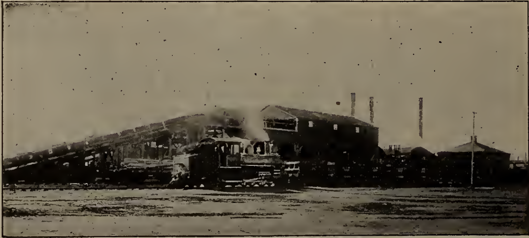
COLLIERIES AT WESTVILLE, NOVA SCOTIA.
